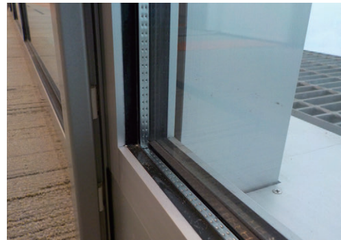
Oizumi Studio main building inner sash Low-E glass windows
